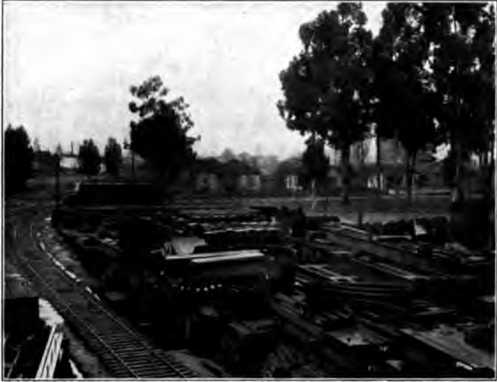
THE BRIDGE-BUILDER LAYS OUT AN ASSEMBLY-YARD FOR GATHERING TOGETHER THE DIFFERENT PARTS OF HIS NEW CONSTRUCTION
